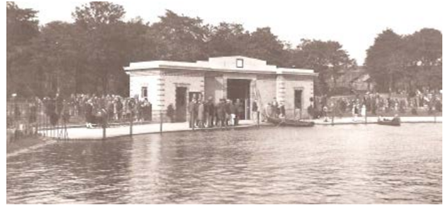
Boat House as constructed
