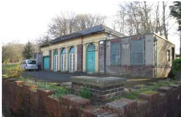
Pavilion as it now stands
